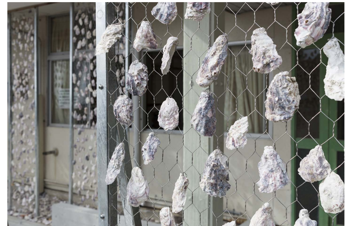
旧沖保育園牡蠣殻スクリーン Oyster Shell Screen of Former Oki Nursery School
